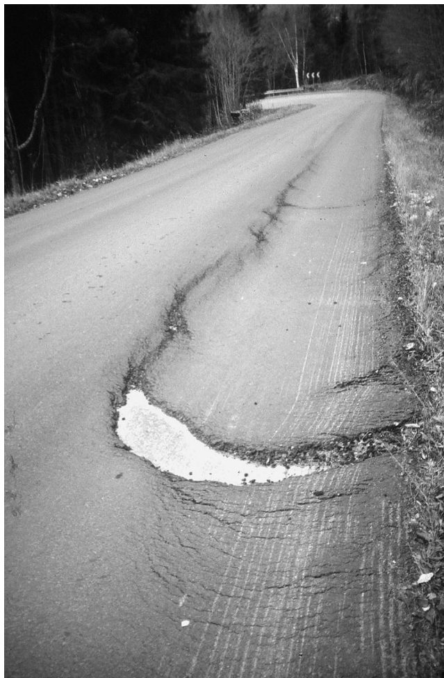
Fig. 1. The asphalted road ca. 500 m east of the E6 junction at Snøan, looking downhill towards the northwest, showing the structures that had developed arising from sinistral strike-slip movement caused by gravitationally induced creep of the 'right-hand' strip of asphalt below the prominent concave-down, rupture scar. The maximum downhill displacement of asphalt at the rupture scar is ca. 35 cm. The white stripes are scratch marks made by a snowplough.
