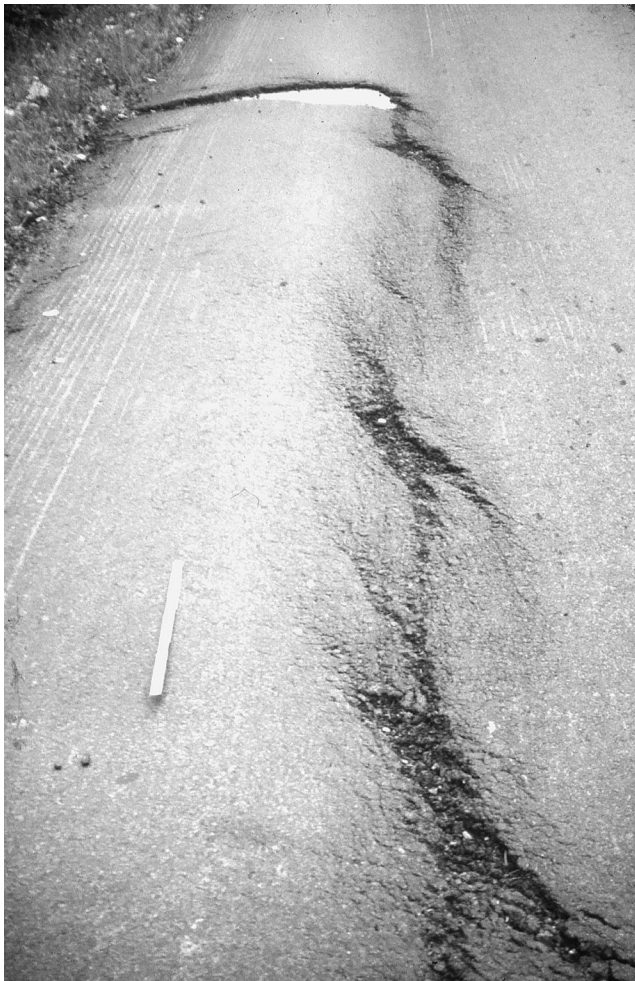
Fig. 3. The same structures as in Fig. 1, but looking uphill towards the rupture scar. The oblique 'faults', at a moderate angle to the sinistral principal deformation zone, and the dark, rhombohedral, transtensional areas akin to pull-apart basins, are easier to recognise as such from this photographic angle.
